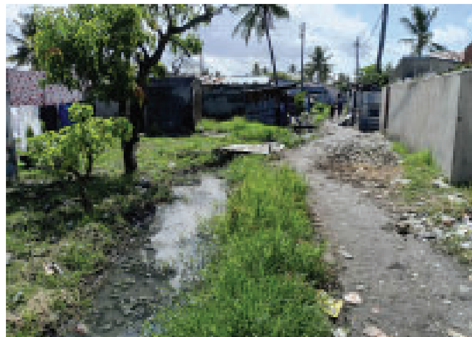
Drainage canal in Goto, a section of the port city of Beira (Mozambique), a neighbourhood close to sea level with precarious drainage infrastructure (picture: Jon Schubert 2023)
